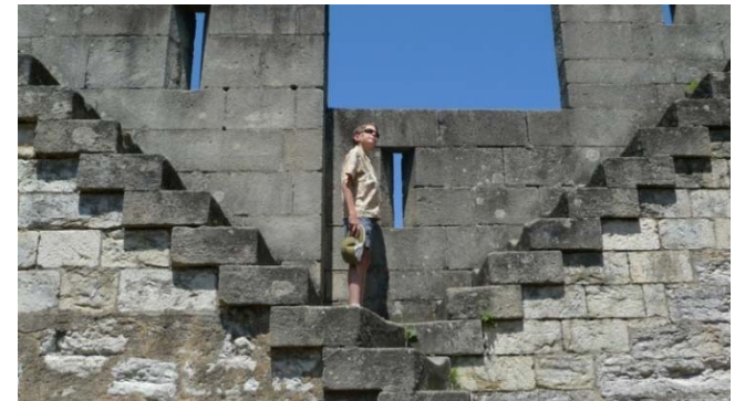
Cool stair up to the battlements on the Pont Valentre
